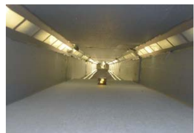
Figure 4-2 (c) Twilight condition (95-135 lx)
