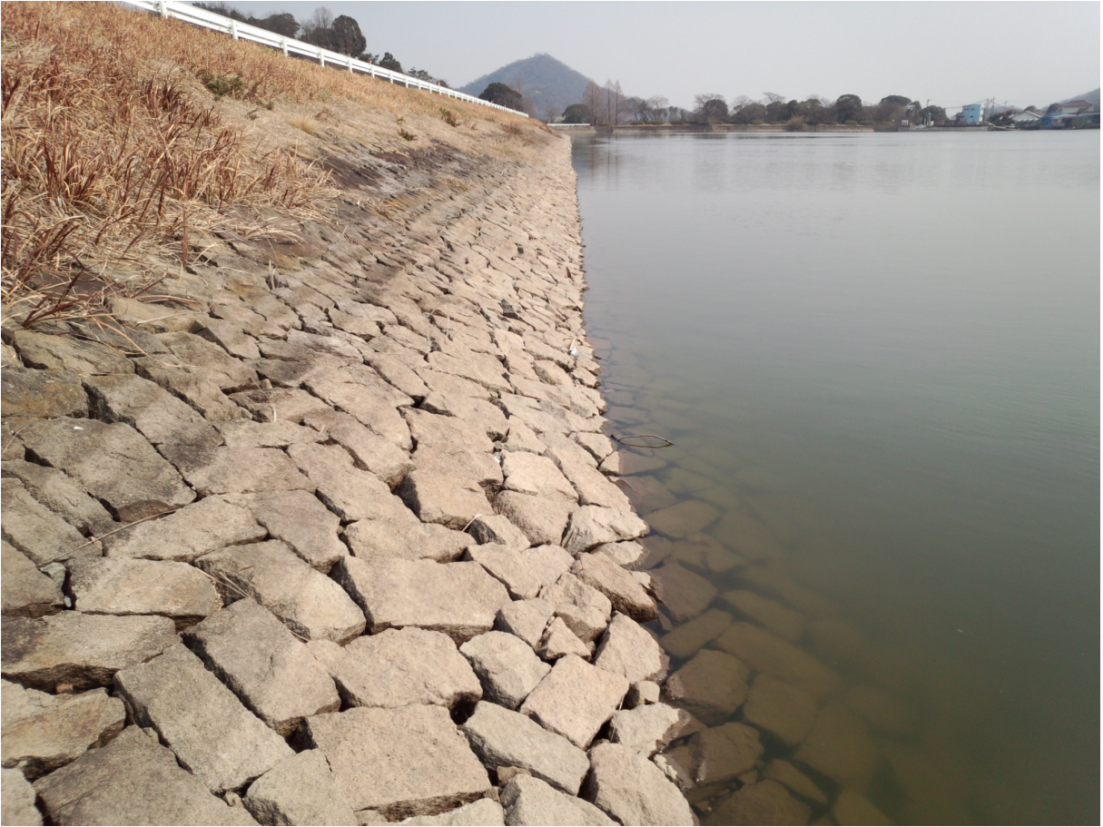
Photo 3.2 Surroundings of Heike (photographed revetment block inside the embankment)
