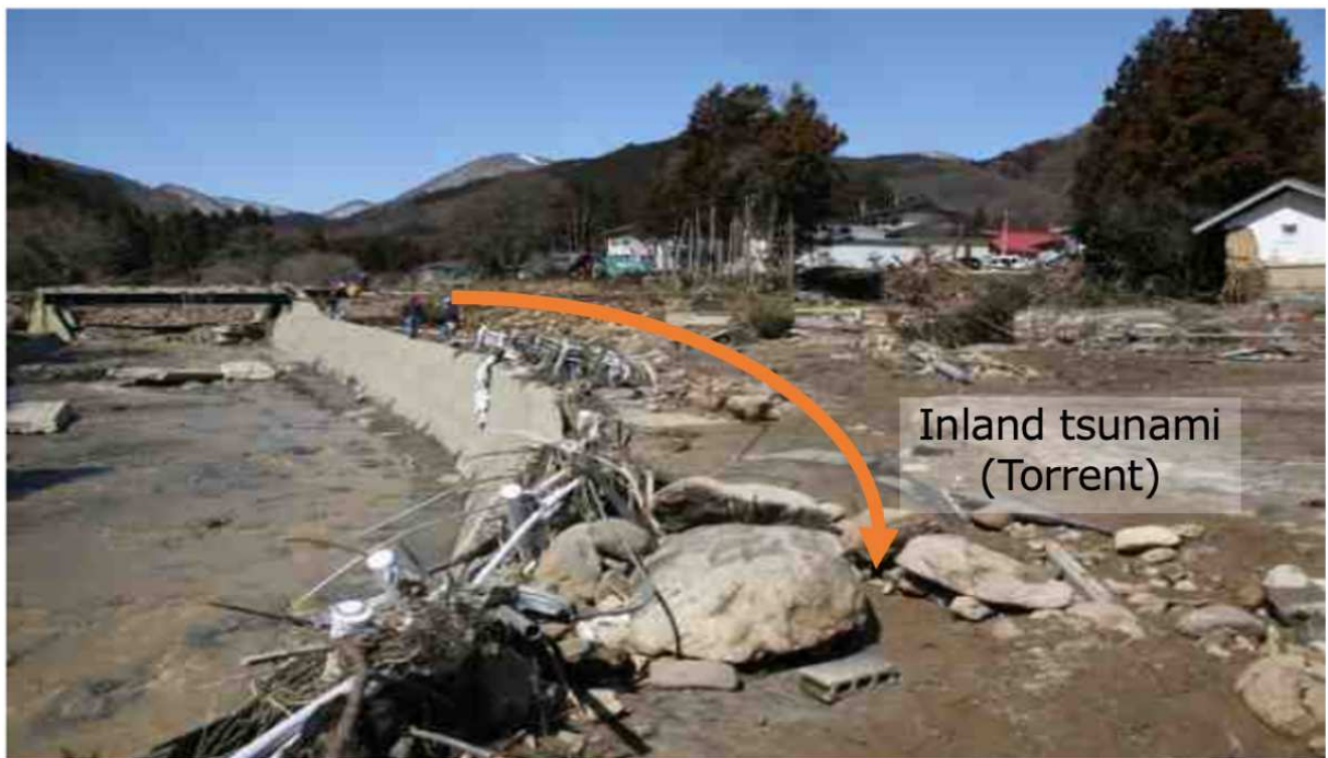
Fig.1.4 Example of damage caused by 2011 the Pacific coast of Tohoku Earthquake (Additional illustration added to the photo excerpted from Sukagawa City data 6) )
